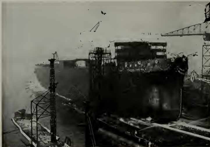
Tonan Maru No. 2 (now sunk) was built as a whale oil factory in 1937 at the Osaka Iron Works for the Nippon Suisen K. K. Gross tons is 19,425 and net tonnage is 13,402. Her length is 534, beam 74 and depth 56.8.
